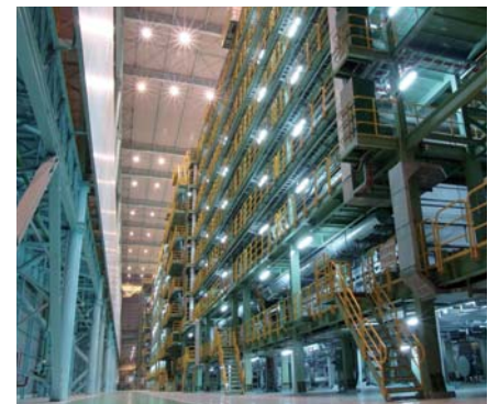
Baosteel & NSC Automotive Steel Sheets Co., Ltd. (BNA)'s Continuous Annealing and Processing Line
