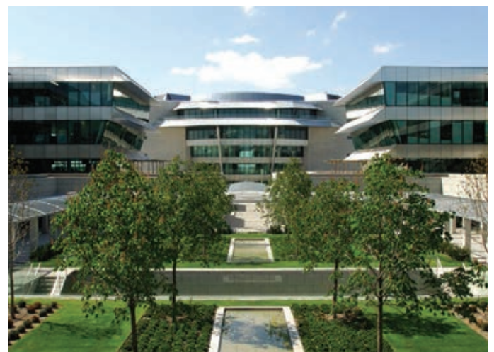
↑ Above Banco Santander corporate headquarters, Madrid.
