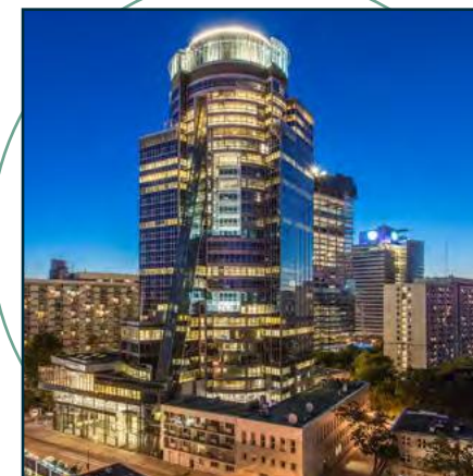
Spektrum Tower, Warsaw
