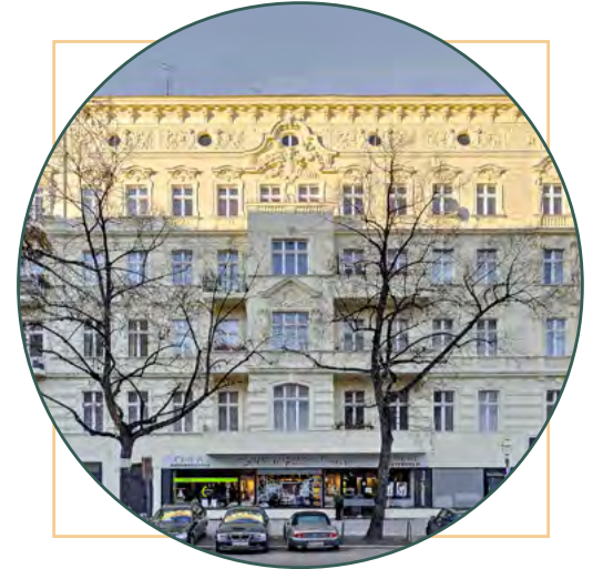
Residential Apartments, Berlin, Germany
