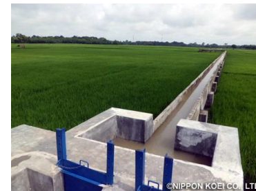
Tertiary canal (Constructed in the Komering Phase 2 Project)
