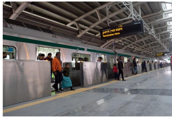
Station platforms with platform doors installed (Photo by DMTCL )
