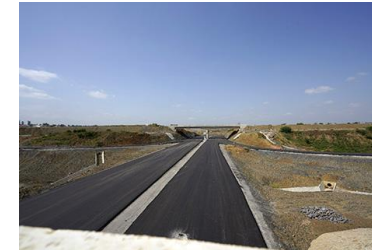
Road under construction
