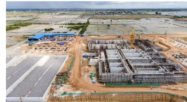
Water treatment plant under construction
