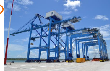
Port cranes constructed
