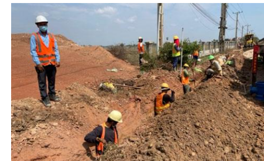
Manual digging for water pipe laying route
