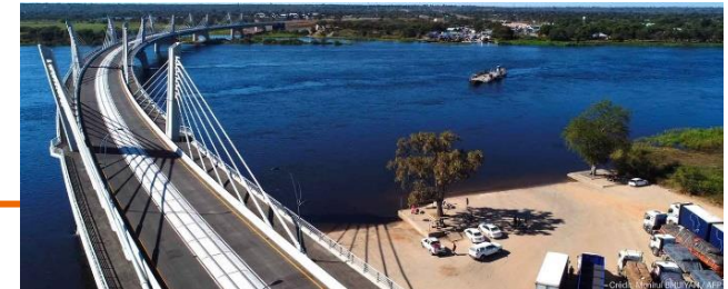
'New Kazungula Bridge' across Zambezi river bordering Botswana and Zambia
