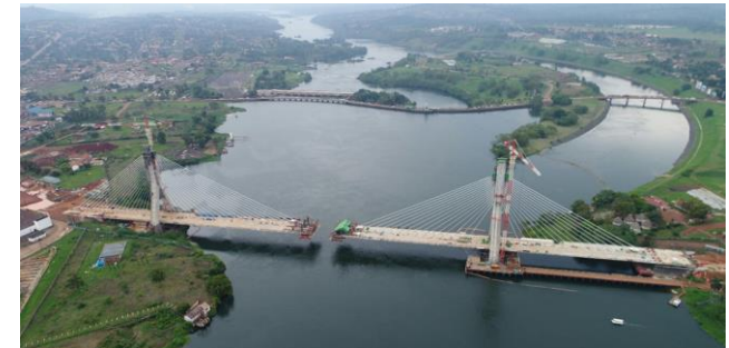
New Bridge Across River Nile
