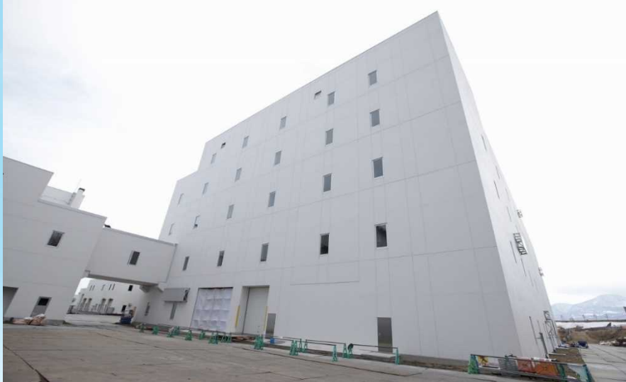
Seibu Sludge Treatment Center
