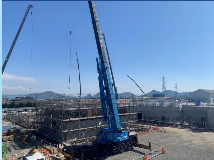
New purification center under construction
