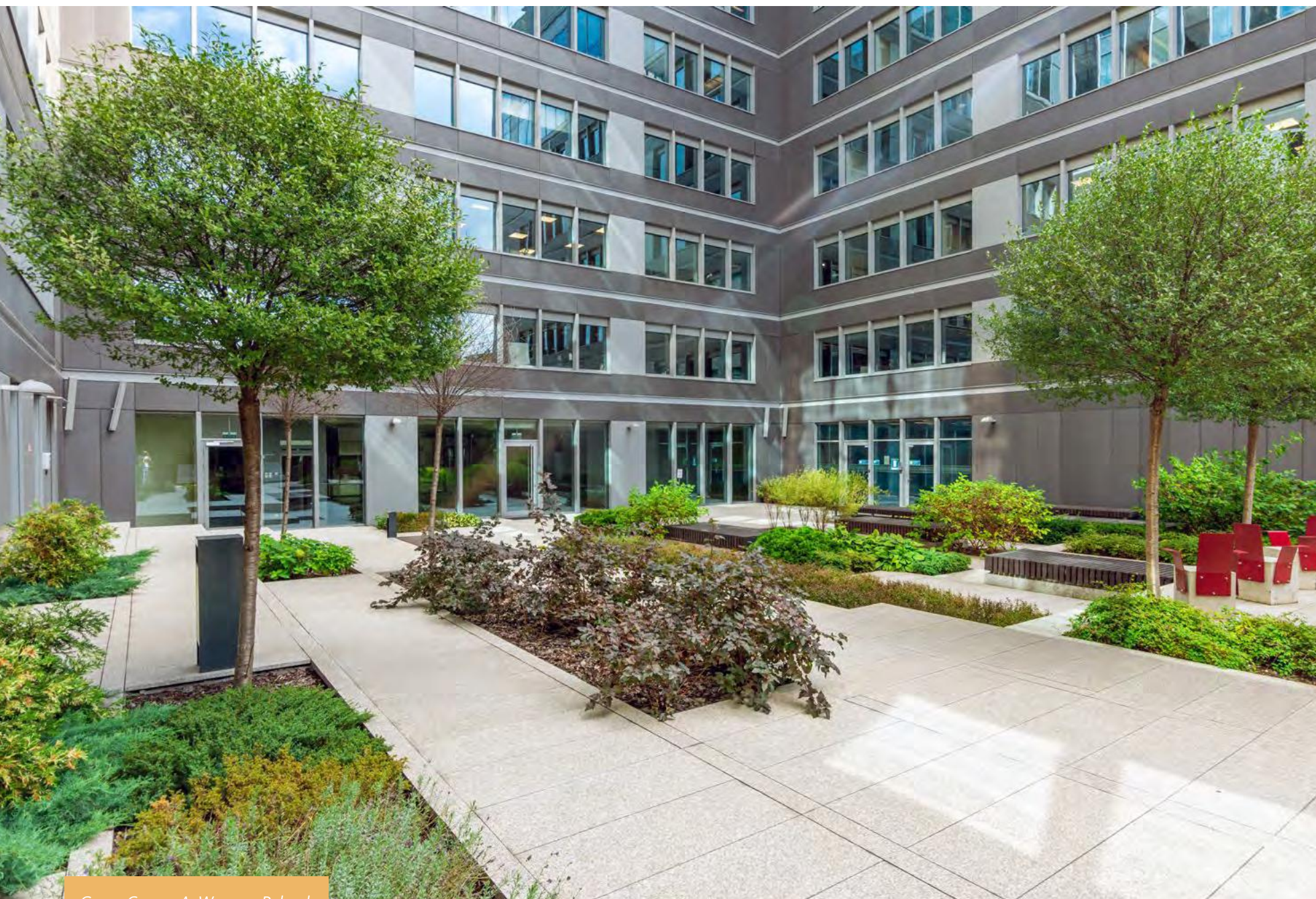
Green Corner A, Warsaw, Poland
